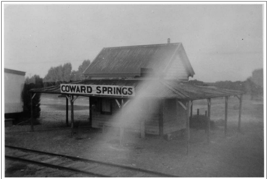
1954 - Coward Springs station building ( George Coop )
